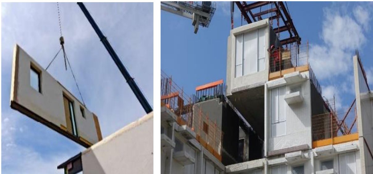
Figure 1. Prefabricated component and MiC lifting process in Hong Kong (ITIB, 2021)
