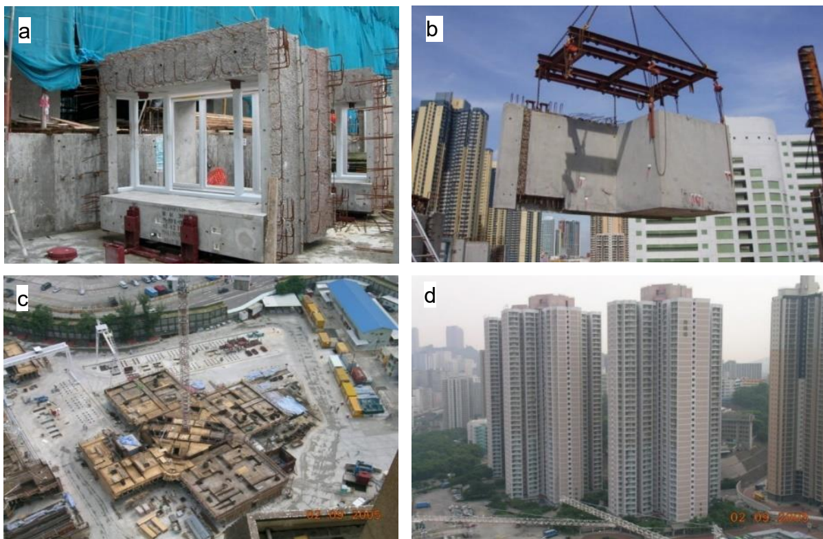
Figure 2. Harmony Block construction project: (a) Precast façade. (b) Precast
