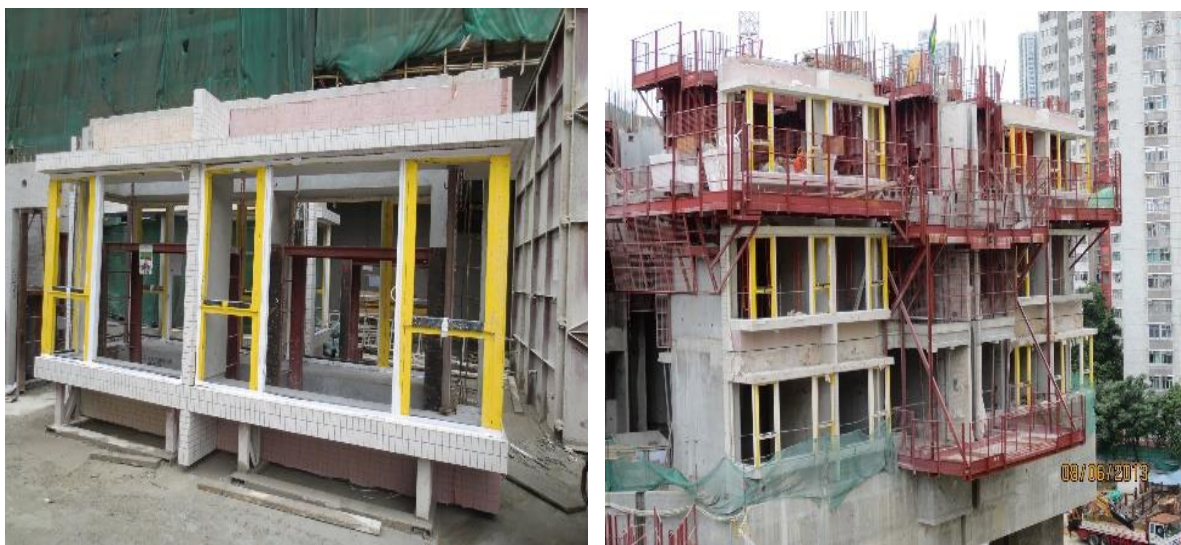
Figure 3. Prefabricated component and construction of Greenview Villailla (HKGBC, 2016)
